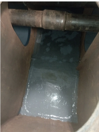
Application of Belzona 1321 on top of Belzona 1311
