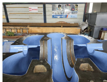
2 coatings of Belzona 1341 completed
