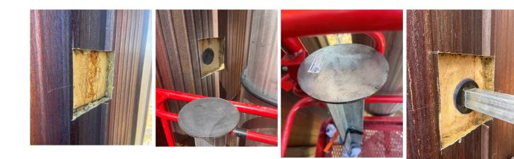
Client identified and marked where support to be bonded on tank exterior. Pipe support and bond area perspiration.
