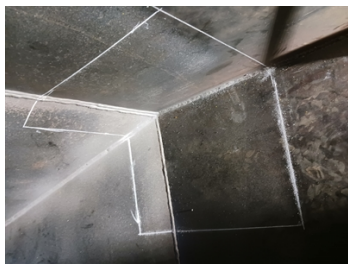
Area laid out for the application of Belzona 1812
