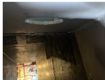
Belzona 1812 applied to the first area
