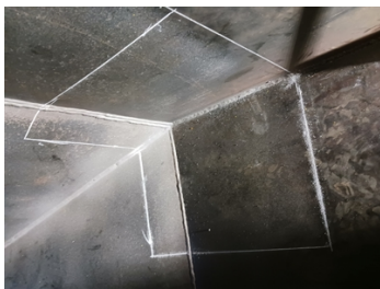
Area laid out for the application of Belzona 1812
