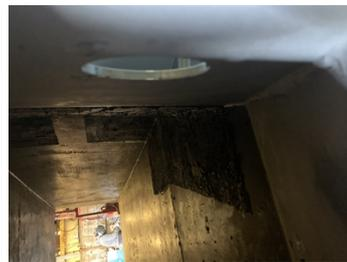
Belzona 1812 applied to the first area
