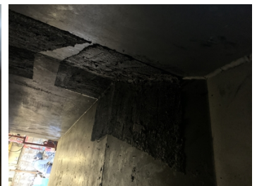
Belzona 1812 applied to both areas on the first chute and hopper
