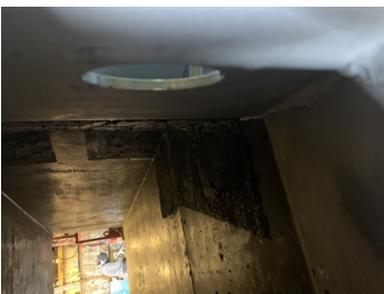
Belzona 1812 applied to the first area
