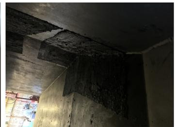
Belzona 1812 applied to both areas on the first chute and hopper
