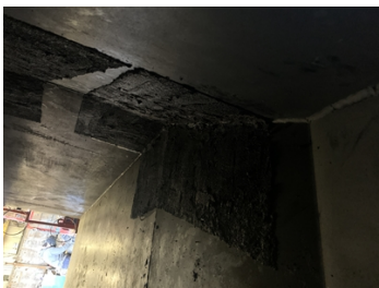
Belzona 1812 applied to both areas on the first chute and hopper
