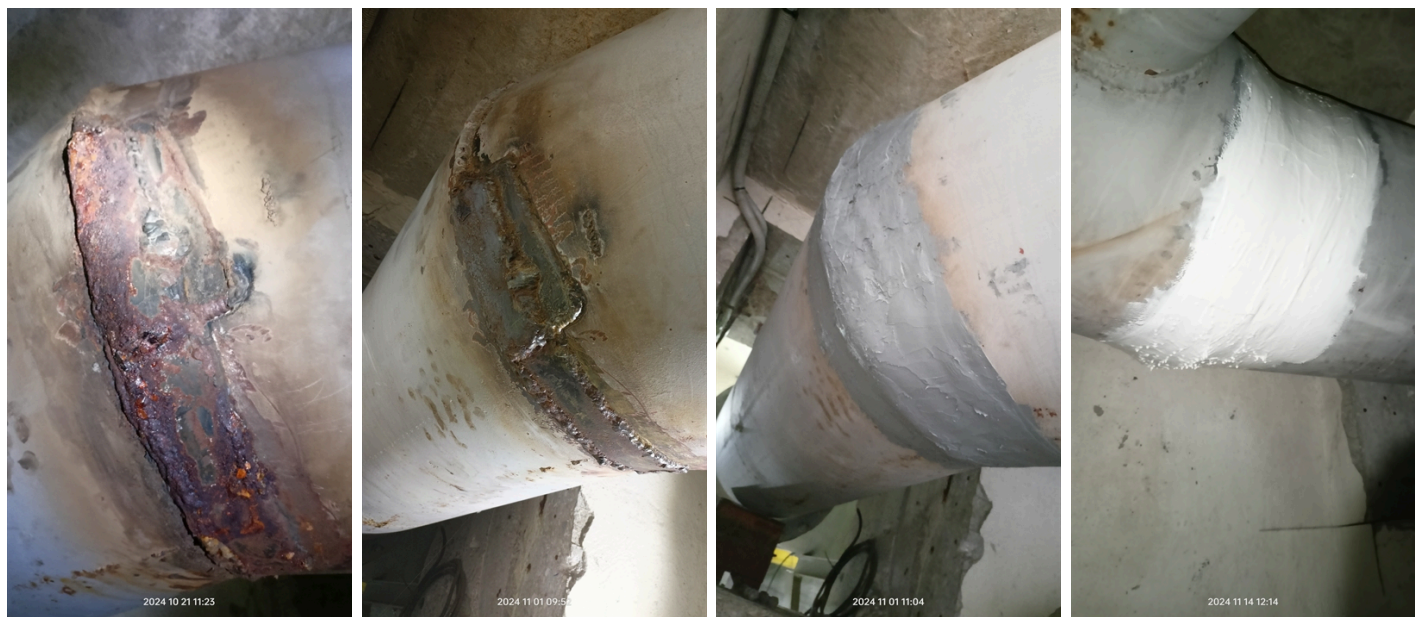
Initial pipe condition illustrating the bonding of the metal pipe with traditional welding.
