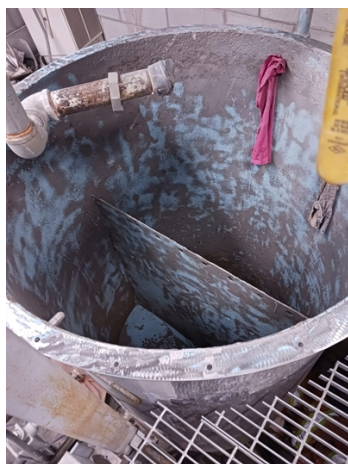
Lining after abrasive blasting.
