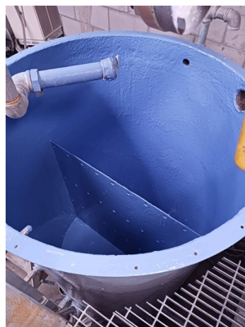
Lining after two coats of Belzona 1341.
