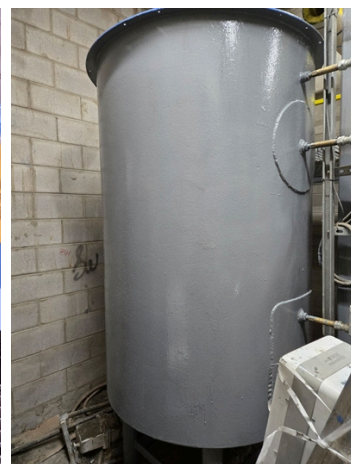
After application of external coating.
