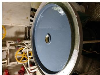
Belzona 1321 applied to the internal chamber lid.
