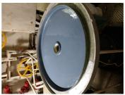
Belzona 1321 applied to the internal chamber lid.
