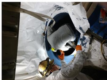
Applying the Belzona 1321 inside the sea strainer.
