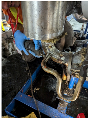
Sealing with Belzona 1221.
