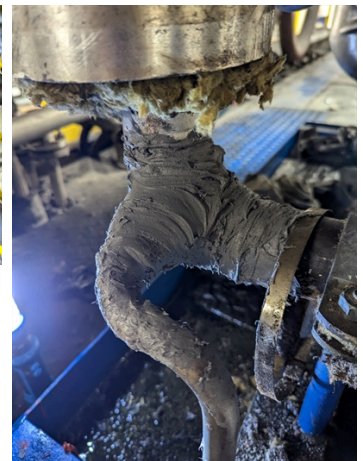
Entire area covered with Belzona 1511.
