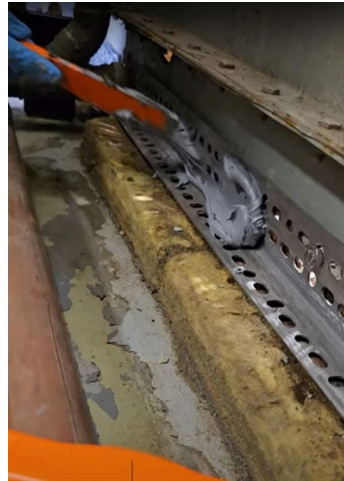
During application of Belzona 1161.
