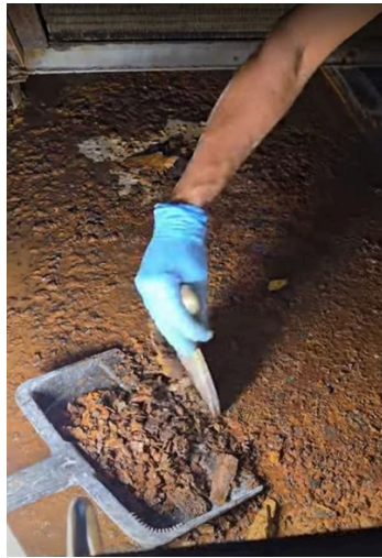
Basin during surface preparation.
