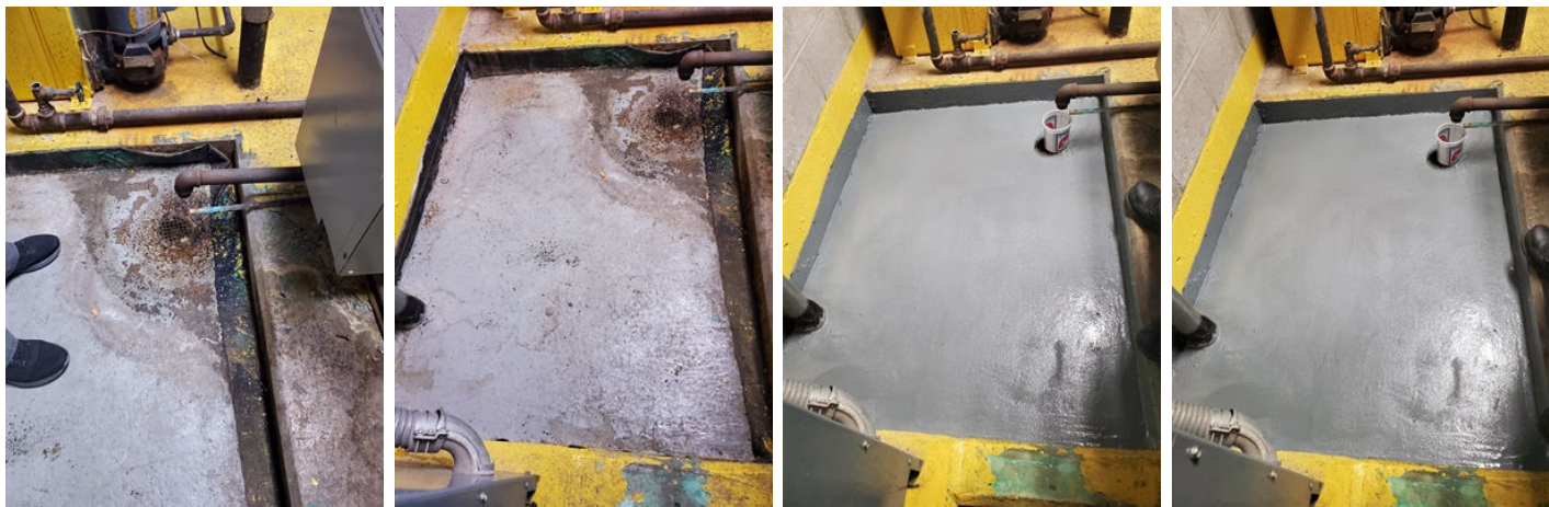
Drain condition before repair with Belzona Drain condition before repair with Belzona Final application of Belzona solution Final application of Belzona solution
