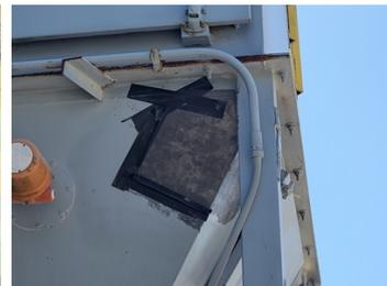
Plate bonding completed
