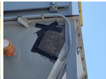
Plate bonding completed
