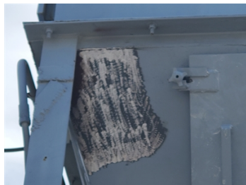
Surface preparation in the equipment
