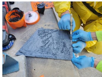
Application of Belzona 1111 on the plate
