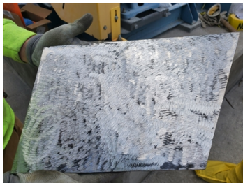
Surface preparation in the plate
