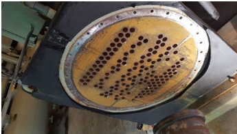
Tube sheet section damaged.
