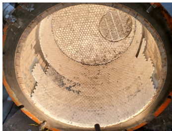
Application of Belzona 9811 tiles (bonded with Belzona 1511).
