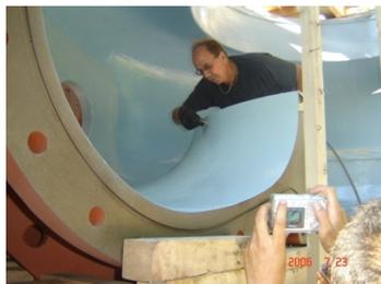
Applicator checking millage of the Belzona 1341 (Supermetalgilde).
