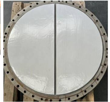
Belzona 1593 application complete.
