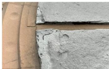
Pitting damage of the cover after grit blasting.
