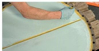
Belzona 1593 application first coat.
