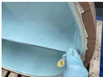
Belzona 1593 application first coat.
