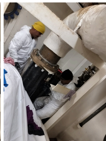
SuperWrap II pipe section being finished.
