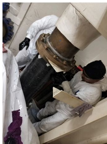
Work and access area for repair SuperWrap II being applied on the pipe section
