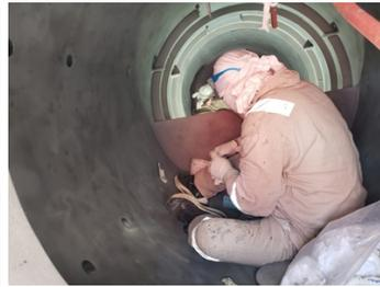
During the application of Belzona 1391T in the vessel, the applicator followed Belzona Know-How System Leaflets TCC-5, TCC-16a, and TCC-16b.
