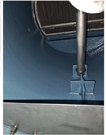
A two-coat system of Belzona 1391T was achieved for the vessel's internal lining.
