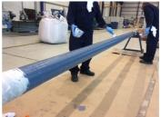
Wrapped with Belzona 9341 Reinforcement Tape, ensuring a 1321 (Ceramic S-Metal) were 6 mm overlap, before the second coat of Belzona 1321 (Ceramic S-Metal).
