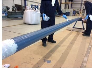
Wrapped with Belzona 9341 Reinforcement Tape, ensuring a 6 mm overlap, before the second coat of Belzona 1321 (Ceramic S-Metal).
