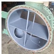
Tube sheet and end cover of the chiller units experienced severe corrosion. Surface was grit blasted and thoroughly cleaned.
