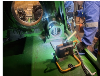
Surface machining after application of Belzona 1111
