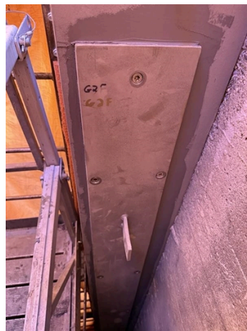
Structure after metal bonding with Belzona 1121.
