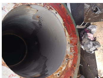
Belzona 1111 application completed.
