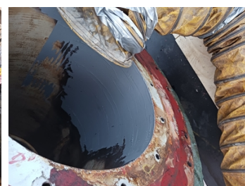
Belzona 1321 application completed.
