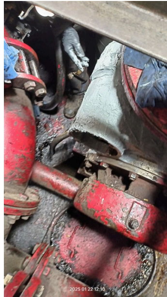
Belzona Super Metal application.
