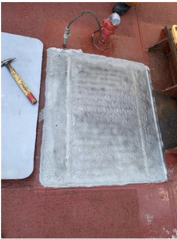
Deck area after abrasive blasting.
