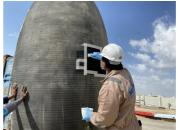
The damaged areas were subsequently repaired and reconstructed using Belzona 2211 (MP Hi-Build Elastomer).
