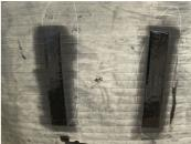
The final layer of Belzona 2111 (D & A Hi-Build Elastomer) was applied for added protection.
