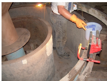
Applying Belzona 1811 (Ceramic Carbide)
