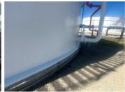
Belzona sealing system being applied. The first layer of Belzona 3111 is reinforced to ensure both mechanical strength and flexibility.
