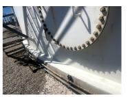
Completed coating with Belzona 3111, forming a seamless and durable barrier against water ingress. An effective and aesthetic protection to extend the asset's service life.
