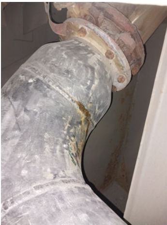
Weakened and leaking areas in the pipelines.
