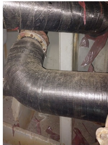
Belzona SuperWrap II has been applied on DN300 pipelines.
