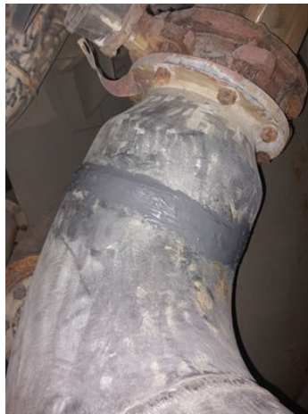
The leaks were repaired by with Belzona 1212.
