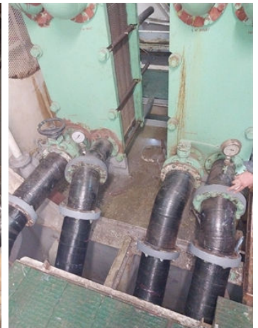
Belzona SuperWrap II has been applied on DN200 pipelines.
