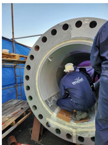
The first coat of Belzona 1391T was applied to the newly fabricated valve
