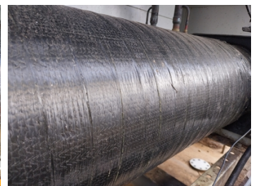
All layers and bespoke ends applied and revisited 3 months on. The customer is totally happy, with no leaks and completely dry floors and dry machinery,
