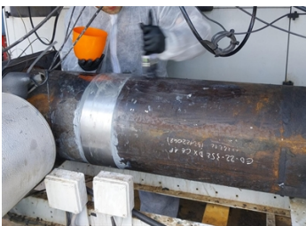
Showing one of the end anchor points bonded to the tube with Belzona 1161
