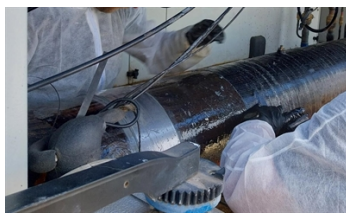
Wrapping the tube after wetting out the tube and composite wrap
