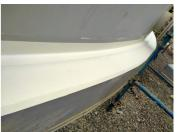
Exposure to harsh environmental conditions can compromise the seal around the annular plate, allowing moisture and air to infiltrate the area.
