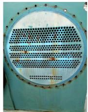
The tube sheet and end cover of the chiller units suffered from severe corrosion, leading to a notable reduction in operational efficiency.
