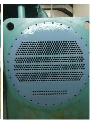
Belzona 5821 was applied as a two-coat system to protect the tube sheet and end cover from corrosion and erosion.
