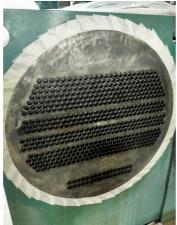
Surface preparation and profile Belzona 1121 (Super XL-Metal) testing were carried out using blasting for the end covers and resurface the worn areas. hand tools for the tube sheet face.
