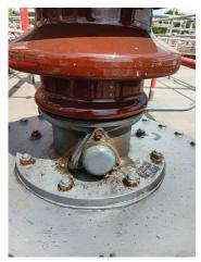
Bushing Flange Bases had been Existing paint removed and identified as leaking oil
