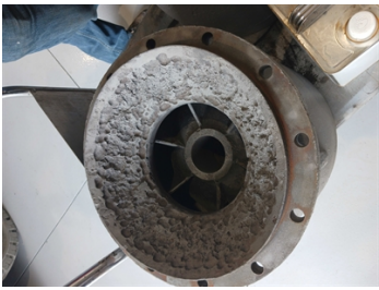
Bowl 1 Corrosion blasted and ready for rebuilding with Belzona 1111
