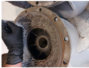
Rebuilding started using Belzona 1111 application by short bristle brush
