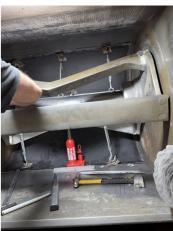
The patch was cold bonded and curing was achieved, ensuring a strong and lasting repair.
