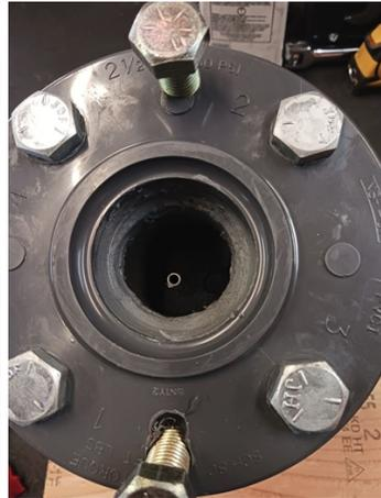
Belzona 1111 placed on flange and former, former bolted to valve body and torqued into place.
