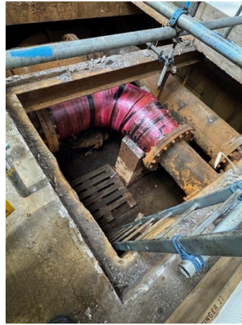
Wrap applied and consolidated
