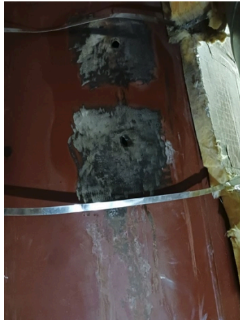
Repair areas on water tank ready for cold bonding of the new plates.
