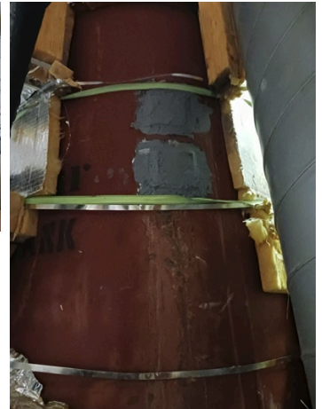
New cold bonded plates applied to tank using Belzona 1111
