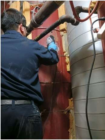
Preparation in progress at corrosion and holed area on water tank.
