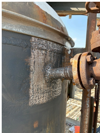
Power tool prep to SSPC-SP 11 using sparkless grinders.
