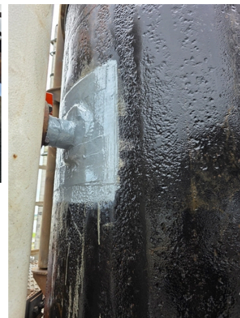
Belzona 5831 used to topcoat system.
