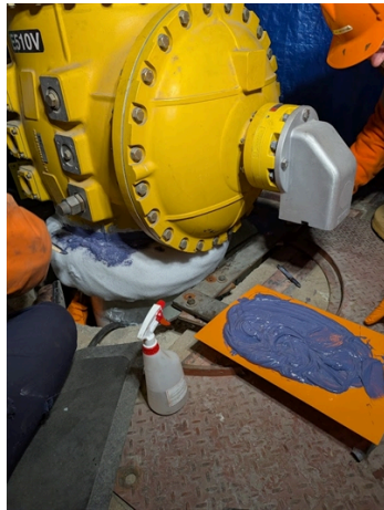
Belzona 7311 being applied onto the Breathing membrane
