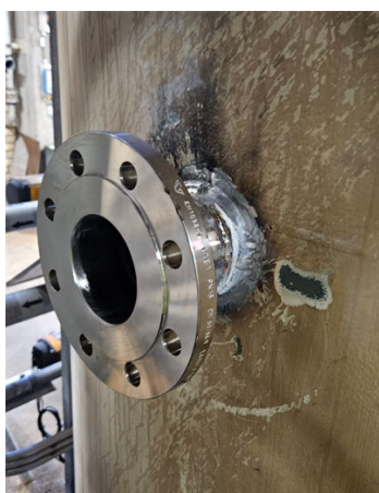
The new pipework is welded and in place
