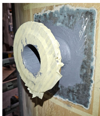
Grouted surfaces with Belzona 1161 to seal around the new weld
