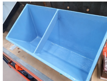
Showing 2nd coat of Belzona 1341 Supermetalgilde
