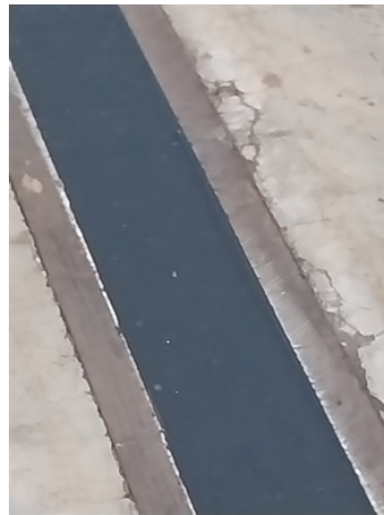
Expansion joint filled and tape removed
