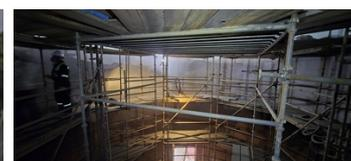
Inspector inspecting the tank for blast ISO 8501-1 Sa 2½ very thorough blast cleaning American Standard near white finish SSPC SP 10 Swedish Standard Sa 2½ SIS 05 5900 d) After blasting, metal surfaces should be coated before any oxidation
