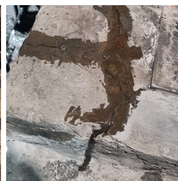
Part way through repairs and concrete stitching, using experienced contractors and Belzona 4151 resins
