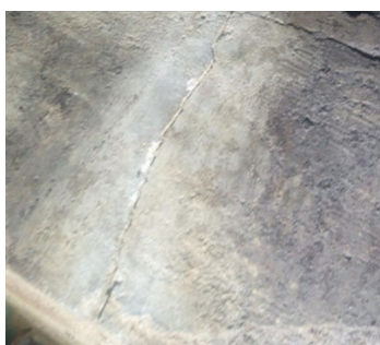
Showing crack to plinth
