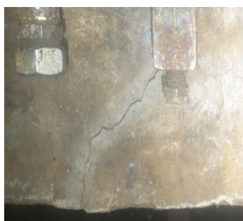
Showing crack on opposite side of plinth
