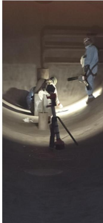
Looking into the Knock out drum for the outside Contractor applying Belzona 1511
