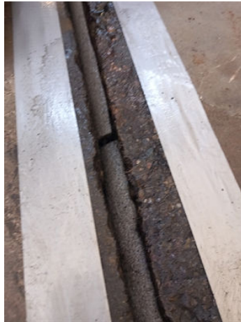
Foam Backer rod installed and Belzona 2911 (Elastomer QD Conditioner) applied
