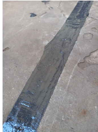
Expansion joint complete and tape removed
