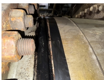
Completion Photo 2: Exterior view of Belzona 2111 applied to the entirety of the expansion joint
