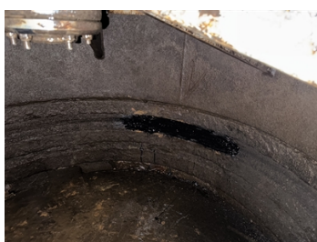
Completion Photo 1: Access into the valve provided a chance to apply Belzona 2911, 2111 directly on the inside of where the leak had occurred. These products applied after preparing the steel+rubber.
